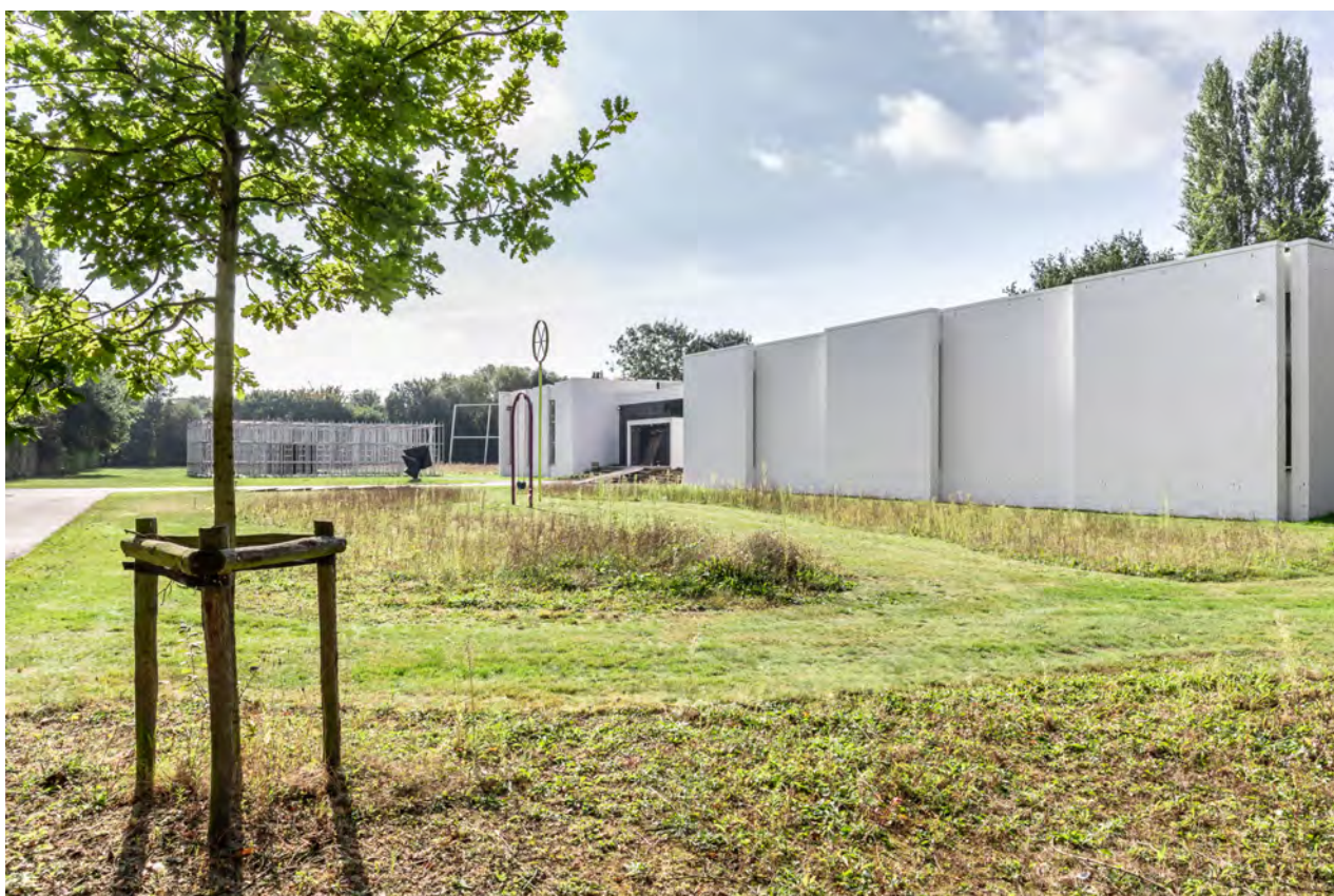
Museum Dhondt-Dhaenens na renovatie, september 2021.
